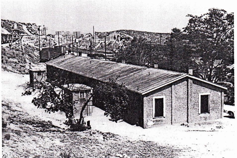
The north and west walls of the concrete bunkhouse at Summit, CA on Cajon Pass show in this view. Also shown next to the bunkhouse are the water closets. Larry Occhiello photo.
